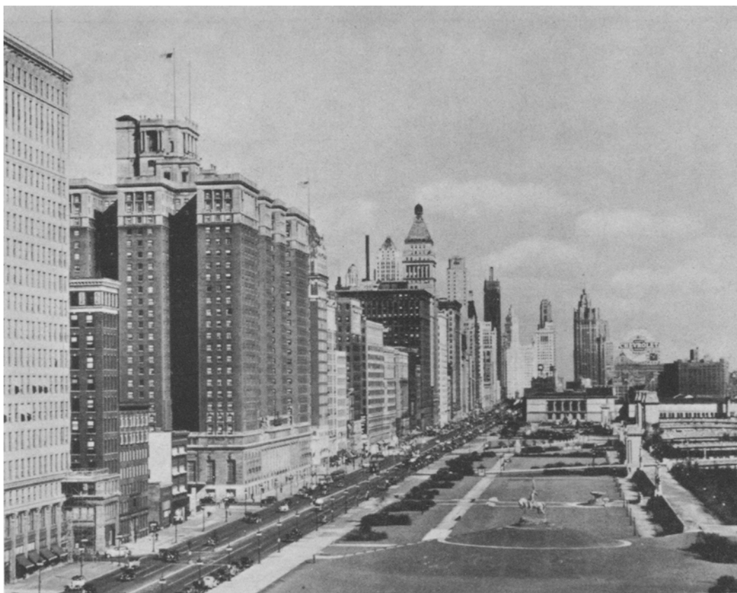
A View Along Michigan Avenue, Chicago
